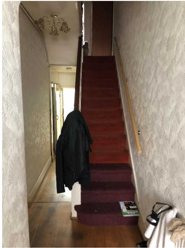
Existing internal staircase
