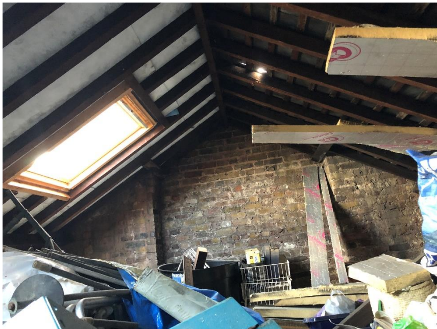
Existing loft space. Non-habitable space.
