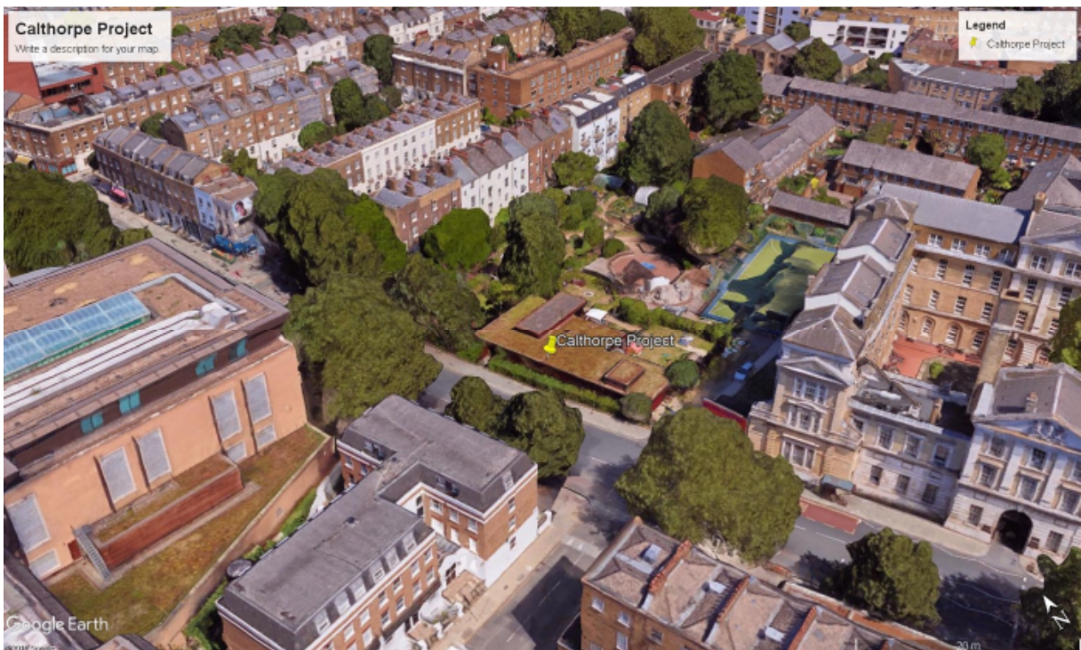
Figure 2: Ariel view of the Calthorpe centre and garden
