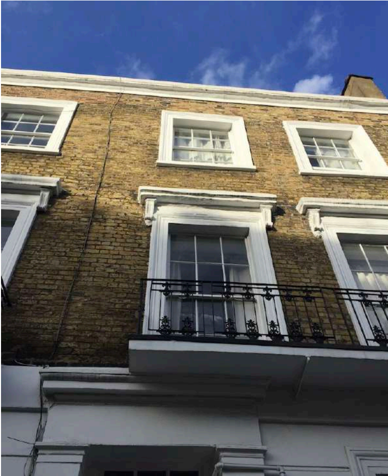
Existing street elevation with stucco detailing, lightwell and iron railings.
