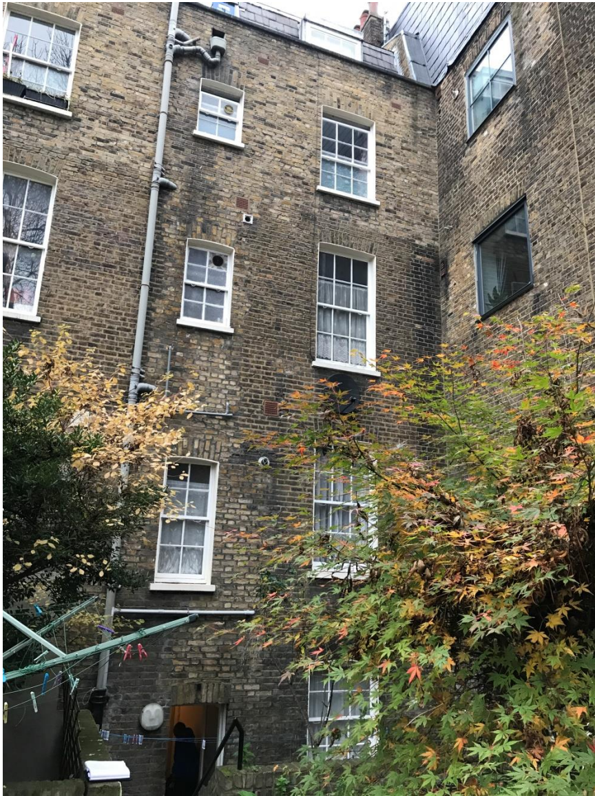
Rear Elevation of No. 29/31 Swinton Street
