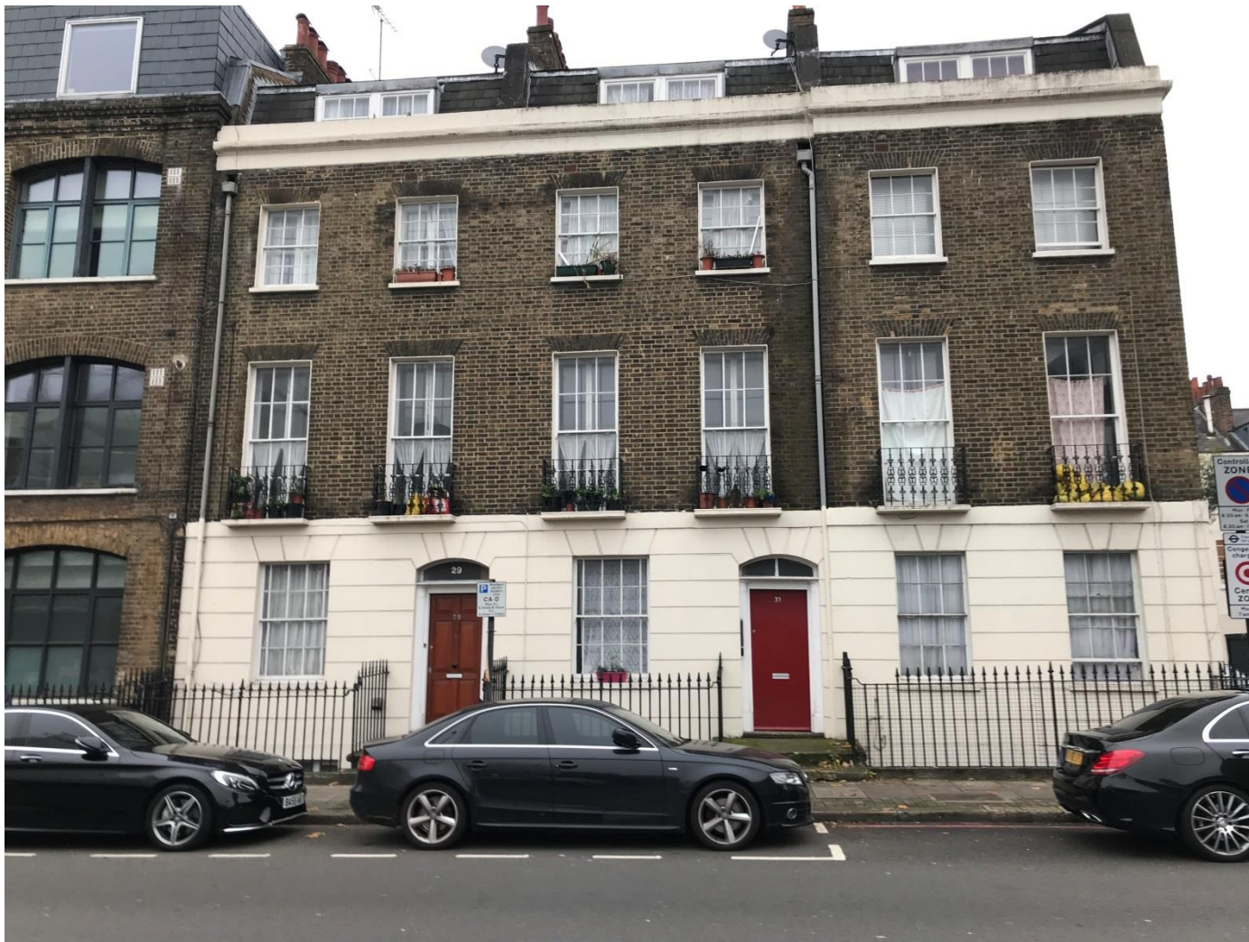
General View of Front Elevation of 29/31 Swinton Street
