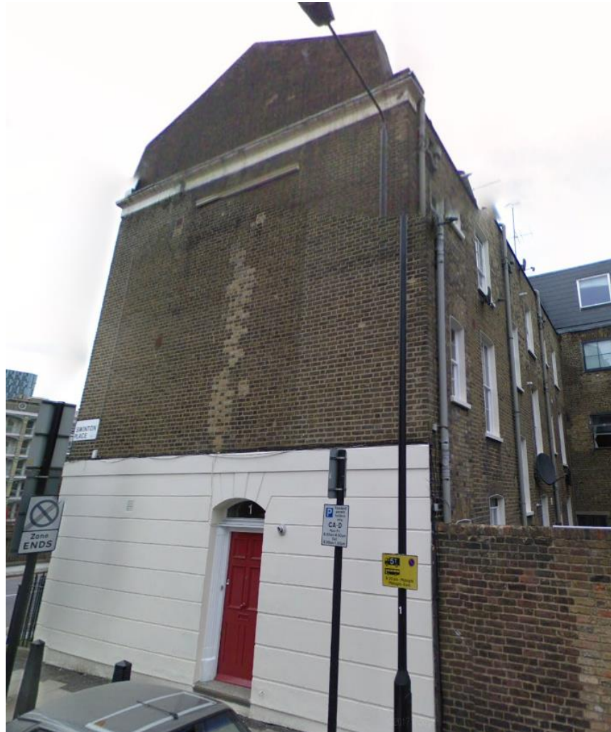
General View of Flank Elevation
