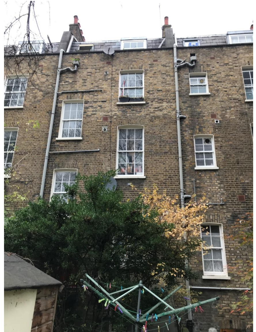
Rear Elevation of No. 29/31 Swinton Street
