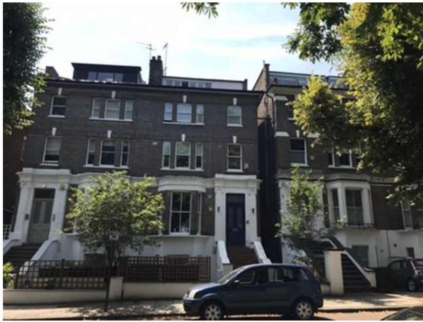
Existing dormer windows 32, 33 and 34 Oppidans Road
