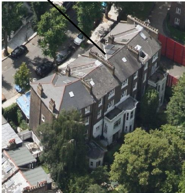
AERIEL VIEW TO REAR OF OPPIDANS ROAD
