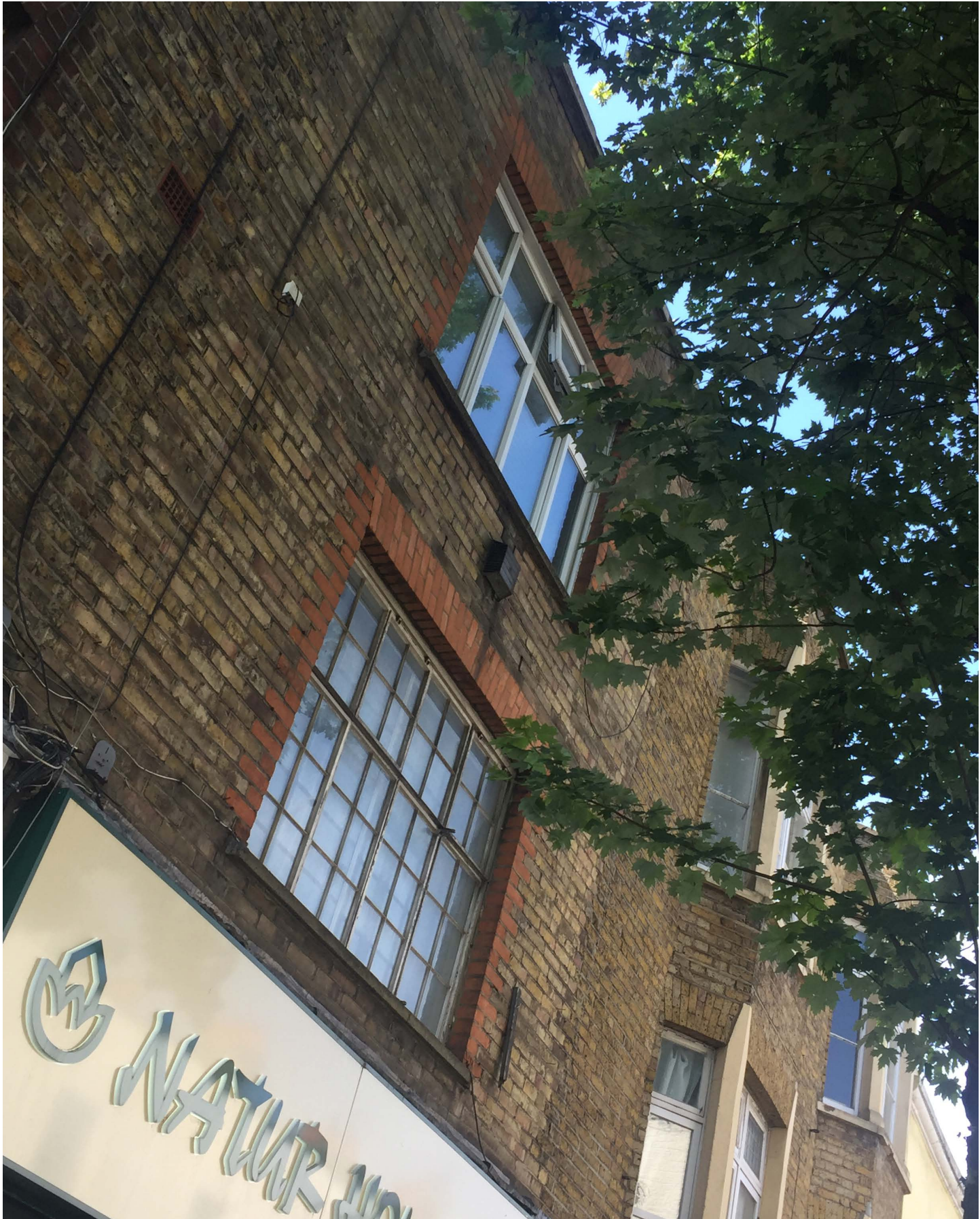
Plastic replacement windows above original Crittal windows in undistinguished building – poor replacement detrimental to the building but characteristic in Parkway.
