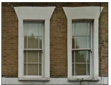
Example of Georgian windows fitted on the property No 112
