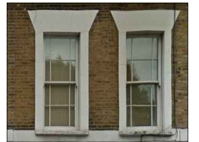
Example of Georgian windows fitted on the property No 112
