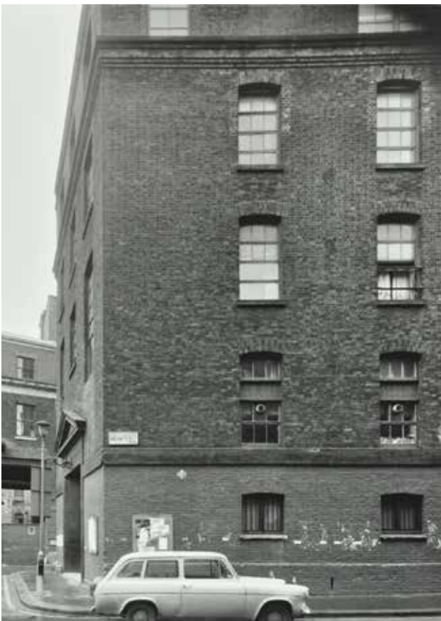
11b. Photograph of the Earlham Street elevation of the Seven Dials Warehouse, 1975 (Collage)
