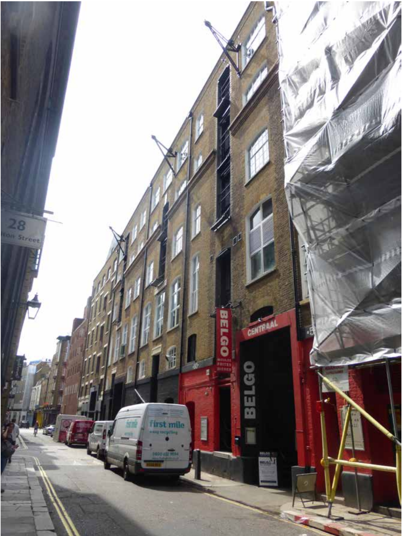
18. Side elevation of the Seven Dials Warehouse facing onto Shelton Street, 2016 (DIA)
