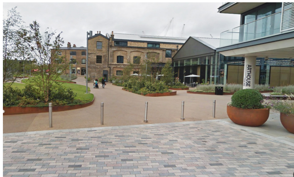
Figure 6: Example of bollard use on Whatf Road, Kings Cross
