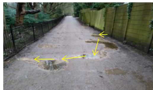
Photos showing permanent trickle of water from pond outfall discharging across Millfield Lane into the Nature Reserve
