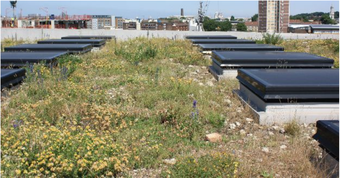
Figure 7: Mature brown roof system
