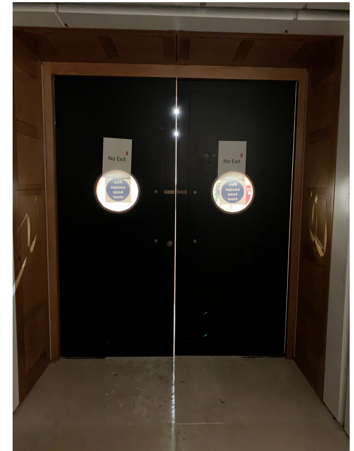
EXISTING DOORS TO GALLERY
