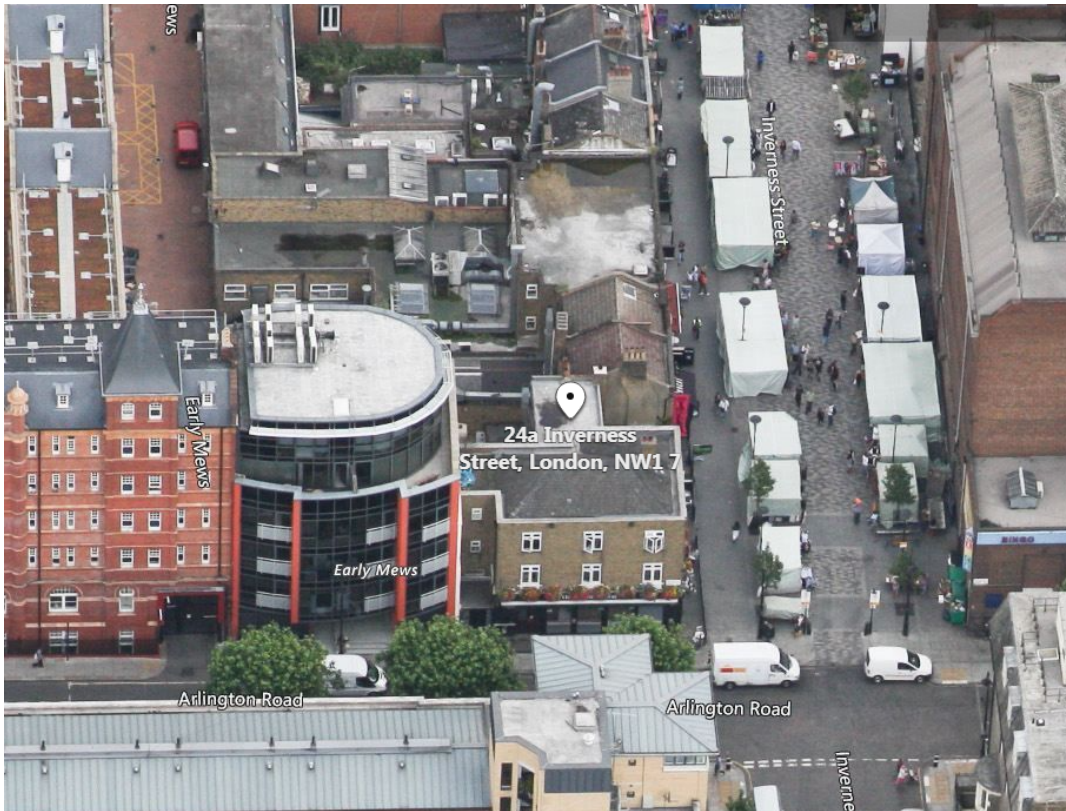
Photo 1 – Aerial view eastwards
