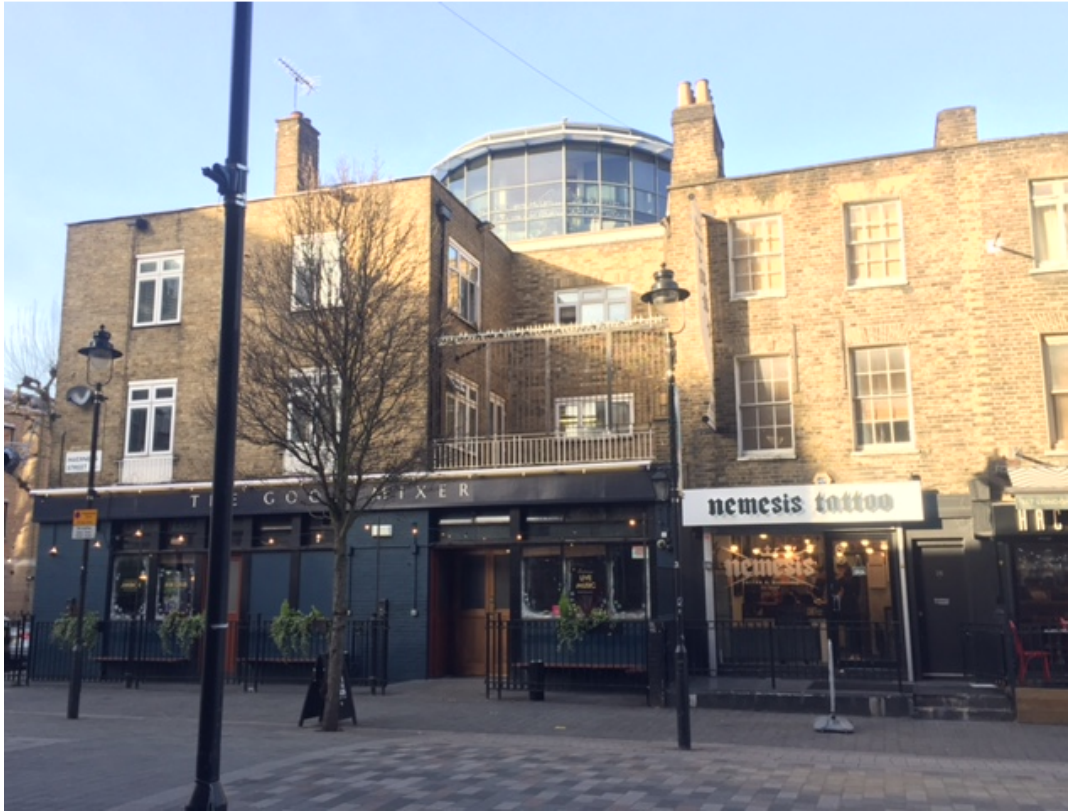
Photo 5 - Full view of Inverness Street elevation
