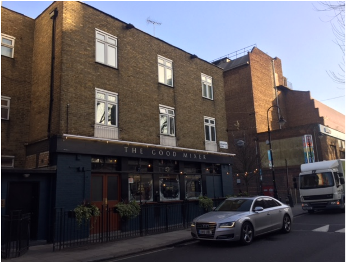
Photo 6 – View of Arlington Street elevation
