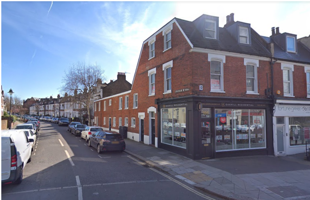
Photo 1 – looking east down Ingham Road
