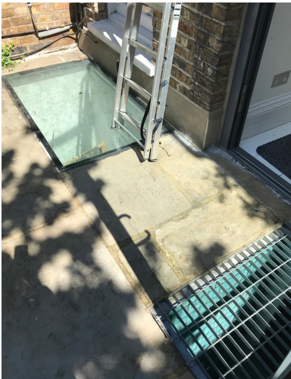
Existing rooflight and gridded lightwell cover
