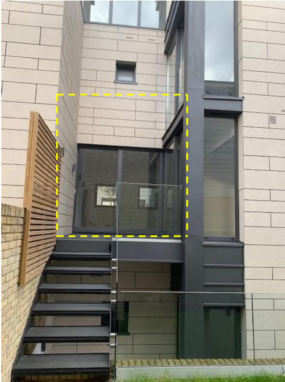
Photo.4 View back towards terrace indicating area of in fill extension.
