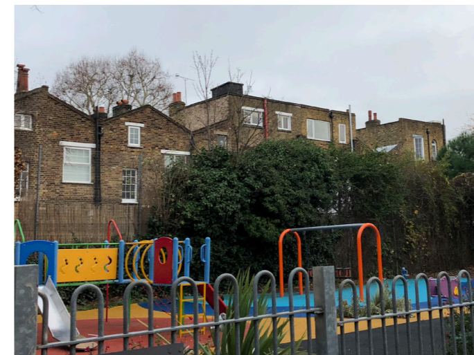
Image 3 - Rear elevation of house on Leverton St.
