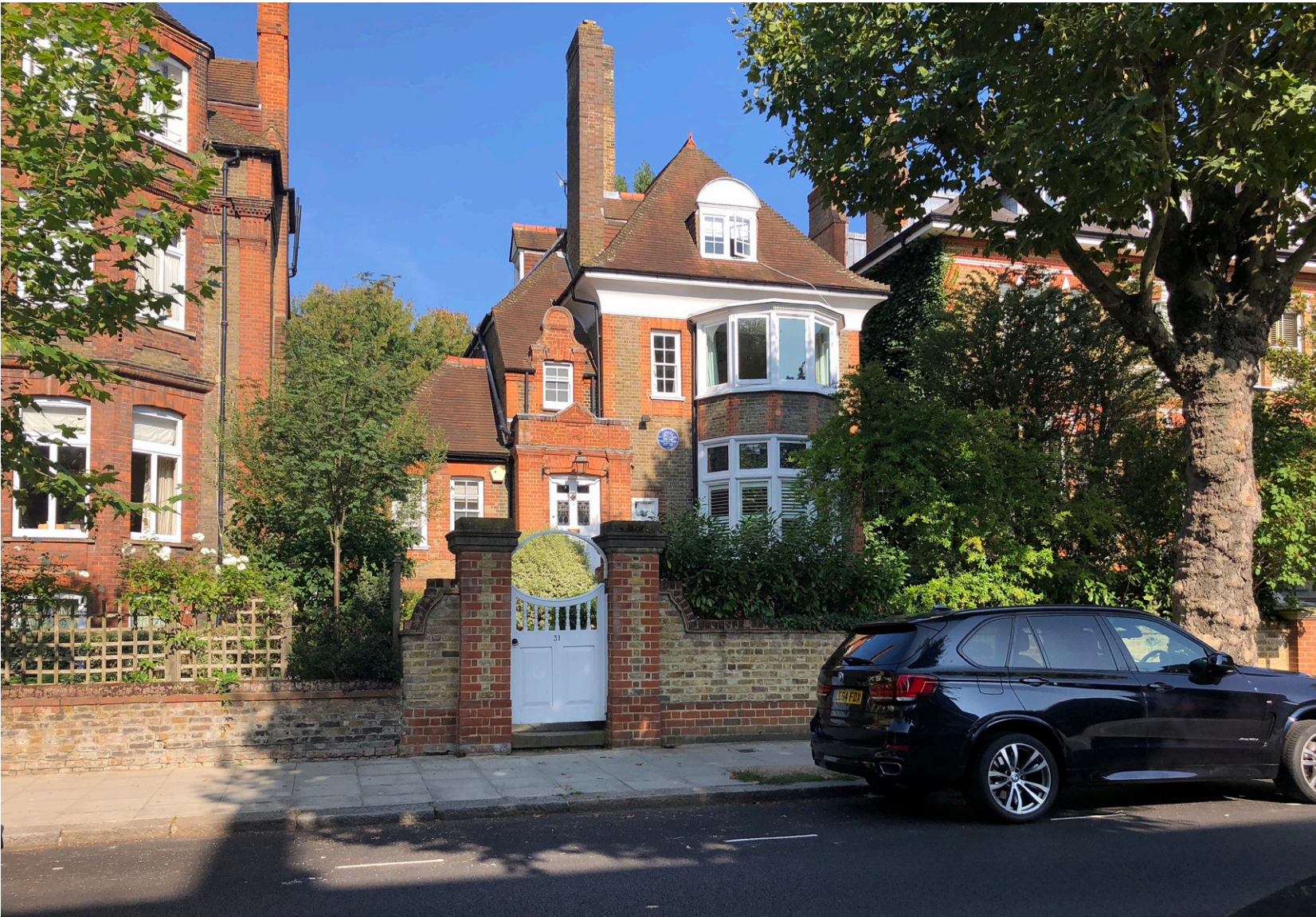
31 Steeles Road front view from the street, 2018
