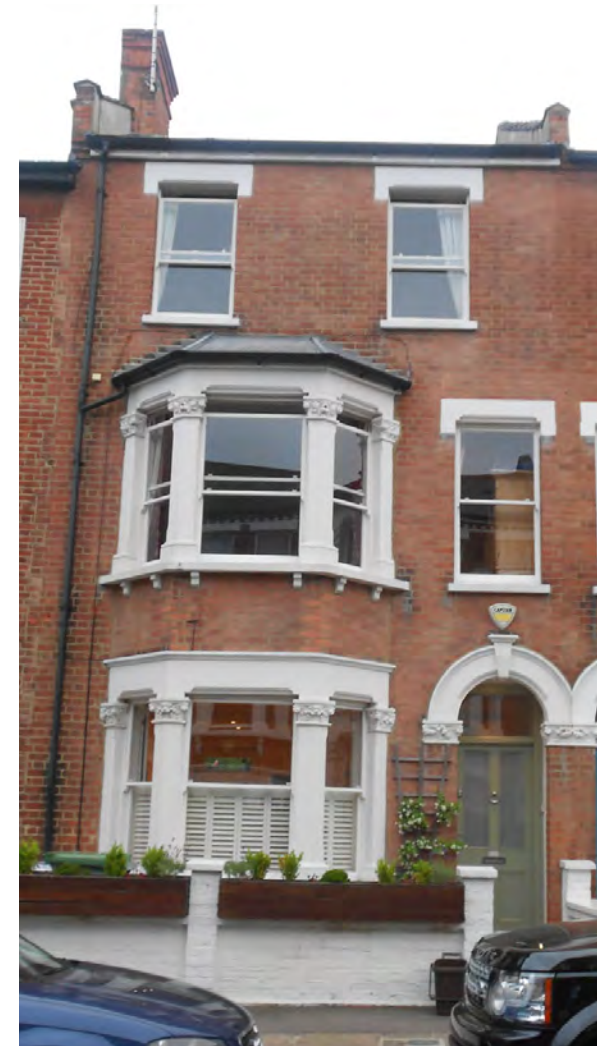
Figure 1.2: PHOTO OF 31 MACKESON ROAD (FRONT)
