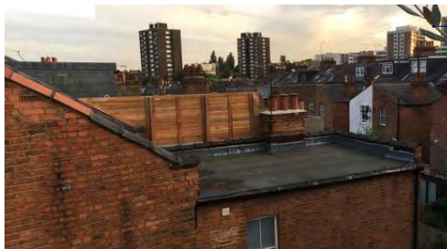
Original configuration of rear flat roof at no. 31 showing unstable chimney stack, now removed - as approved by LB. Camden
