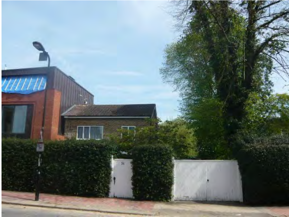
Photograph 1: View of the Site from Redington Road
