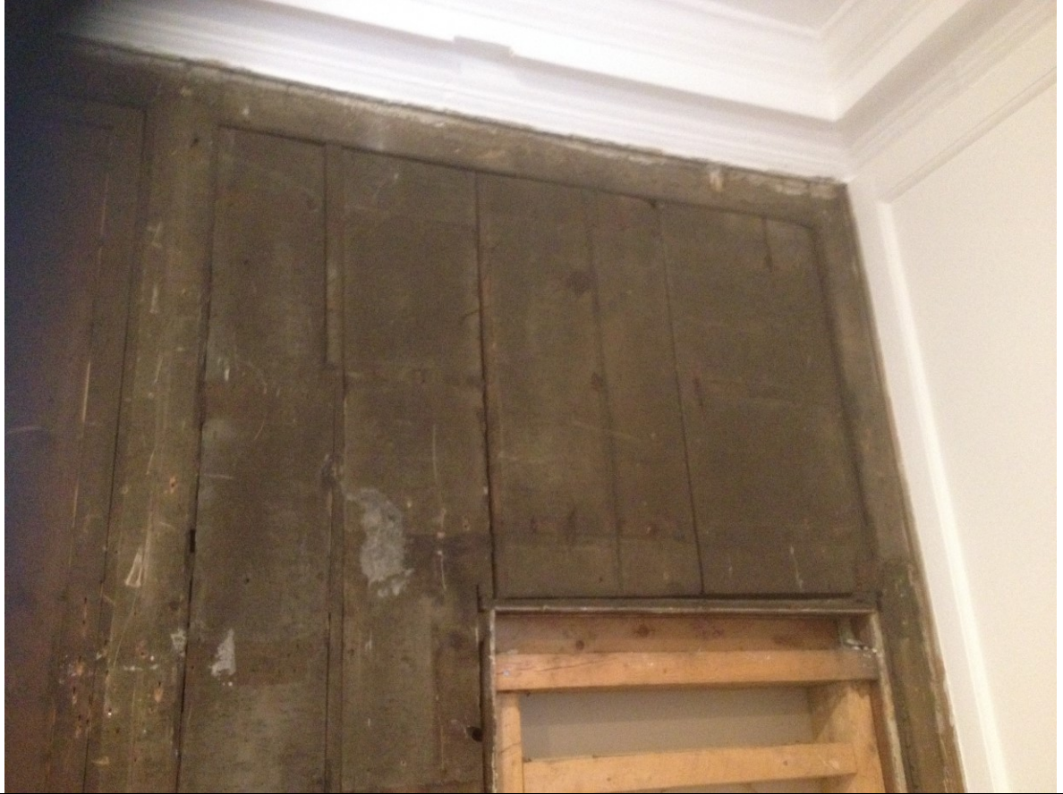
Close up to show plain boarded wall with evidence of fixings for stretched oilcloth (canvas) lining to this side
