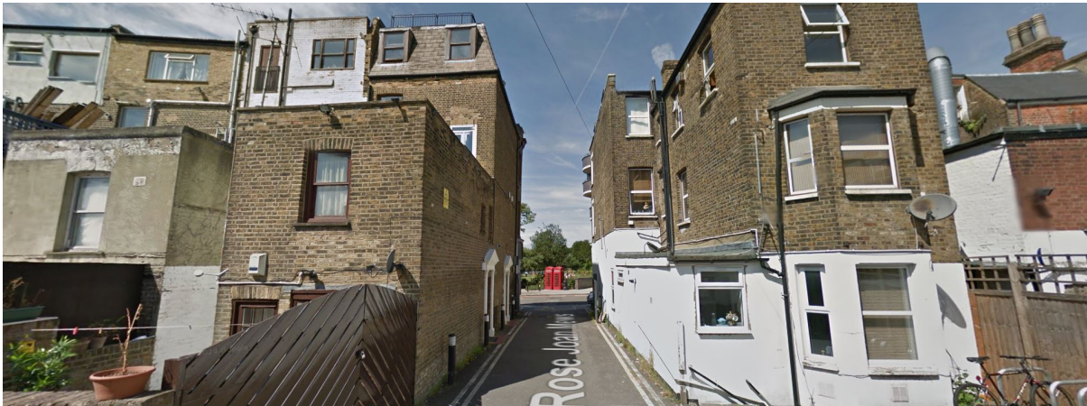
Figure 4 View of rear of Fortune Green Road from Rose Joan Mews (Courtesy Google)
