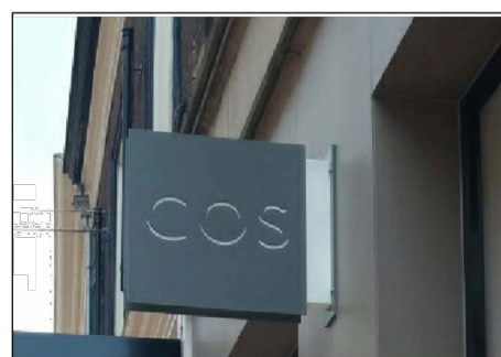
05- Flag sign installed Non illuminated flag sign.
