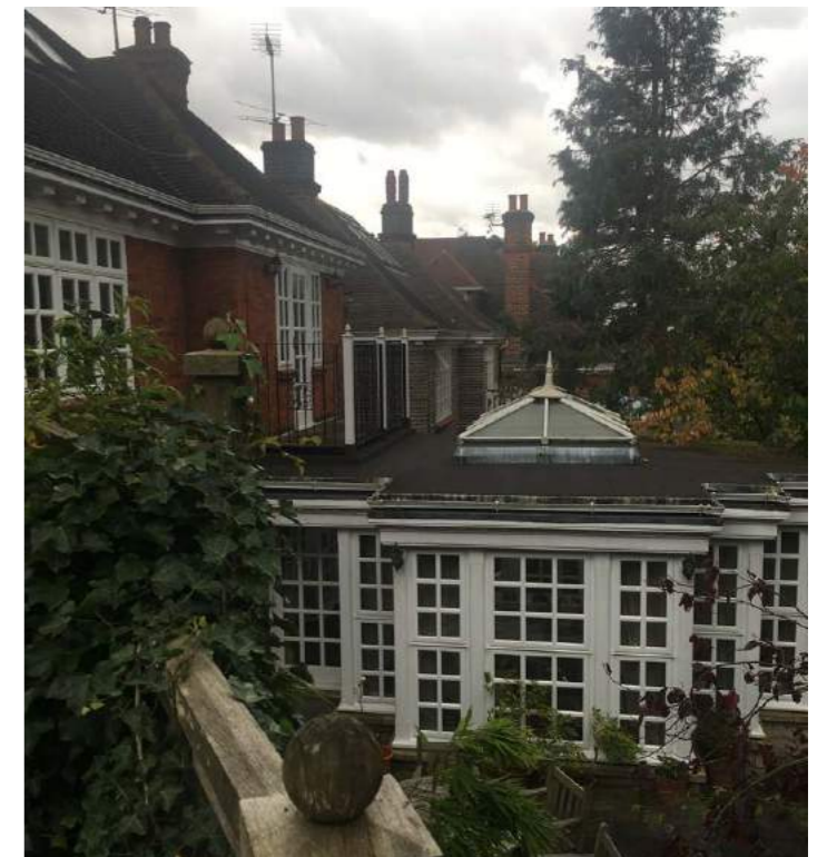
EXISTING REAR TERRACE TO 5 ROBIN GROVE
