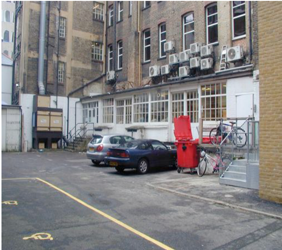
View of parking and delivery area to rear of 18 Chenies Street
