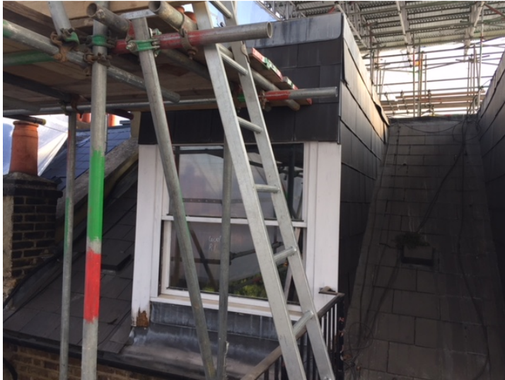
Photo 1 (above): Existing north-eastern rear dormer window
