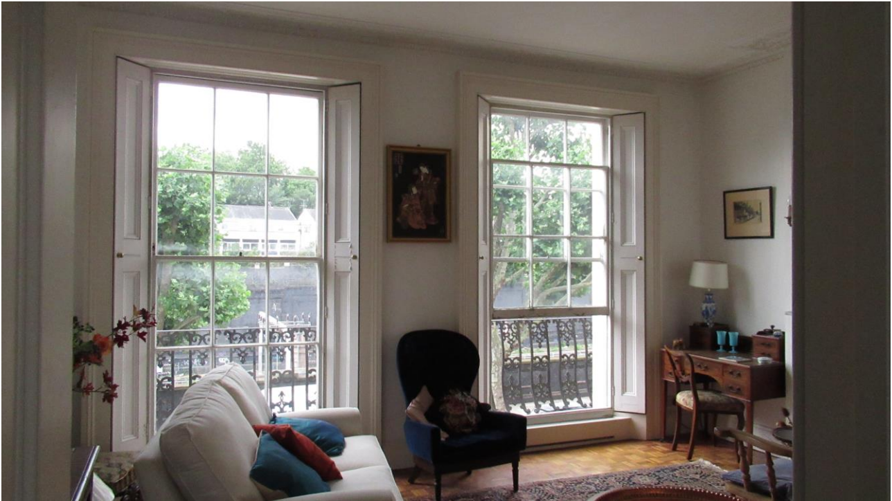
Figure 3: Internal view of windows to first floor
