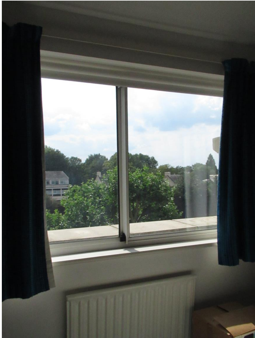
Figure 5: Internal view of window at third floor
