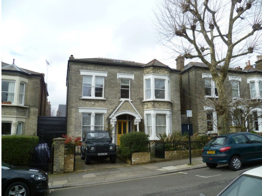
Figure 1: Photo of the front
