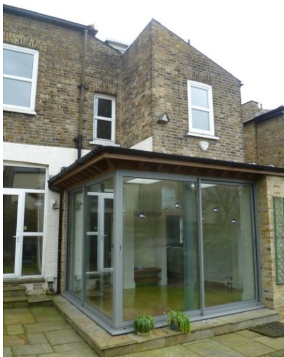
Figure 6: Photo of the 21st Century extension
