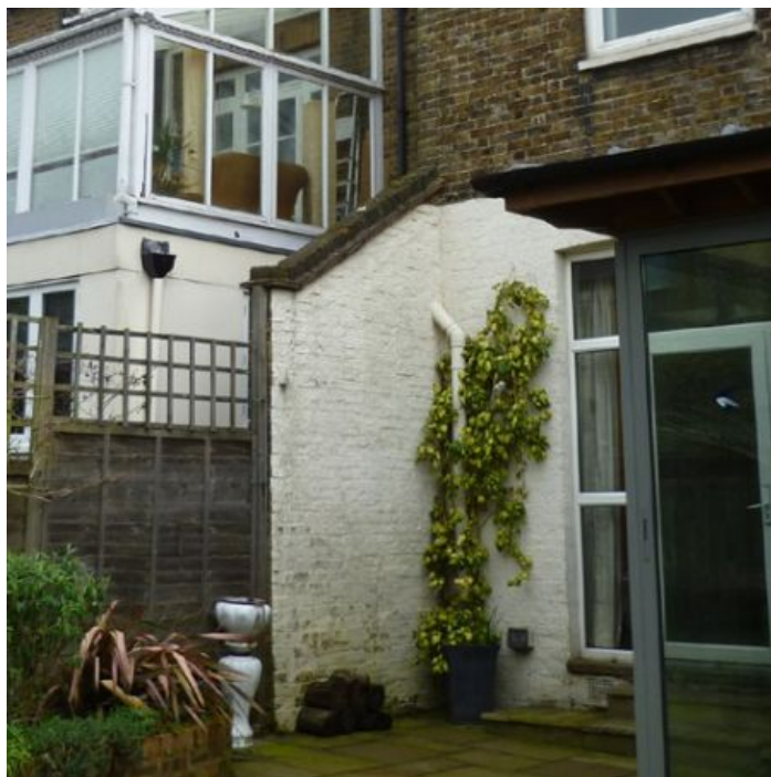
Figure 9: Free standing wall showing extent of original ground floor
