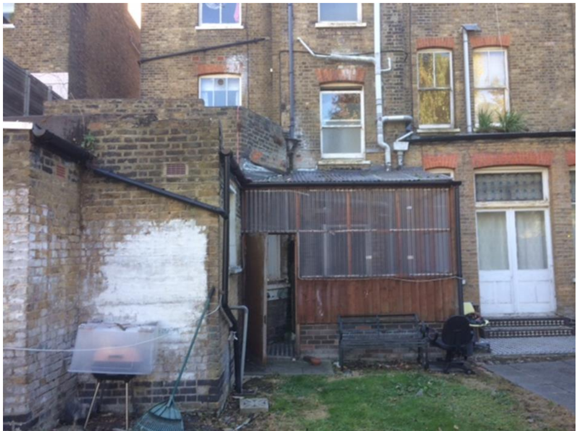
Rear Elevation of 110 Greencroft Gardens
