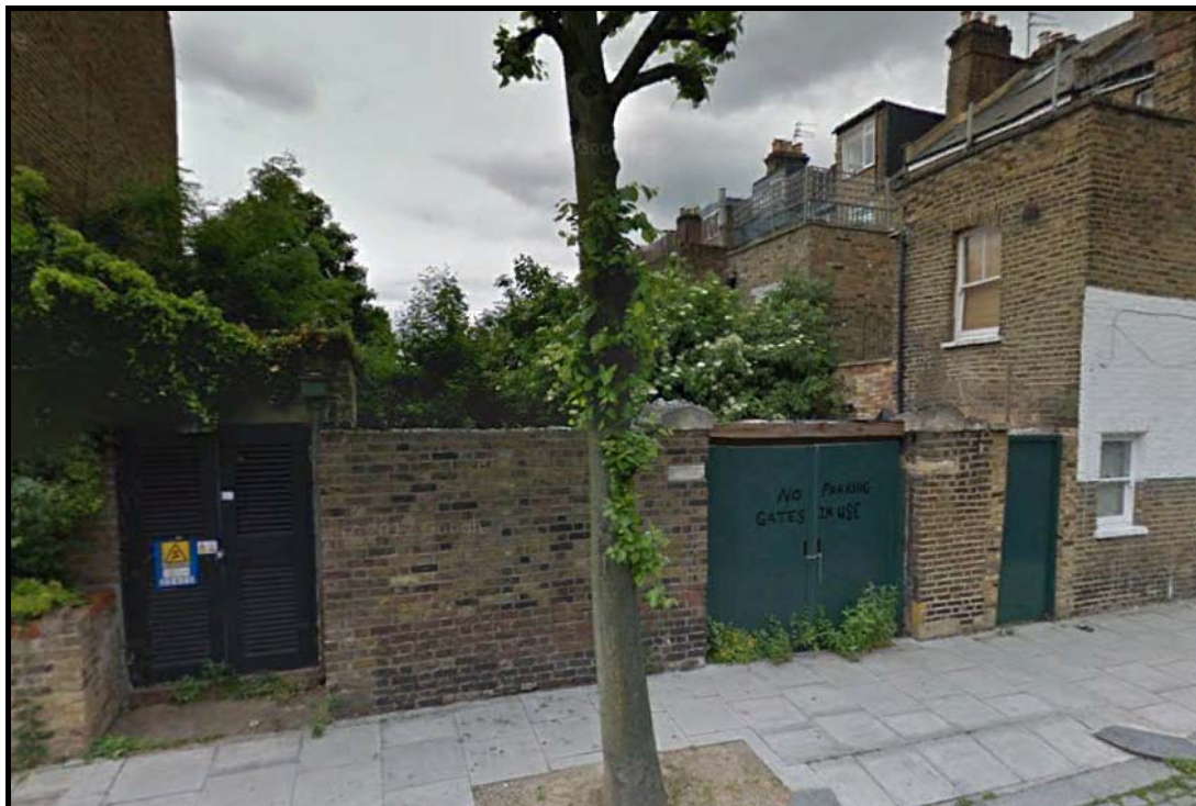
Figure 3 Former Site Façade showing electricity substation
