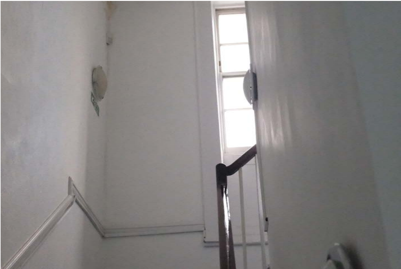
1J. First to Second Floor Stairwell 3060.JPG
