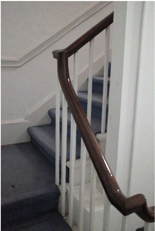
1J. First to Second Floor Stairwell 3059.JPG
