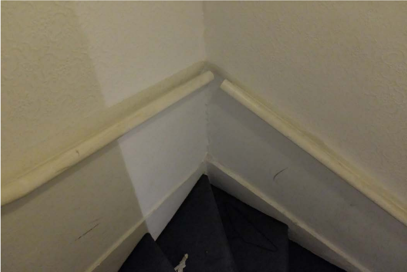
2J. Second to Attic Storey Stairwell 3083.JPG
