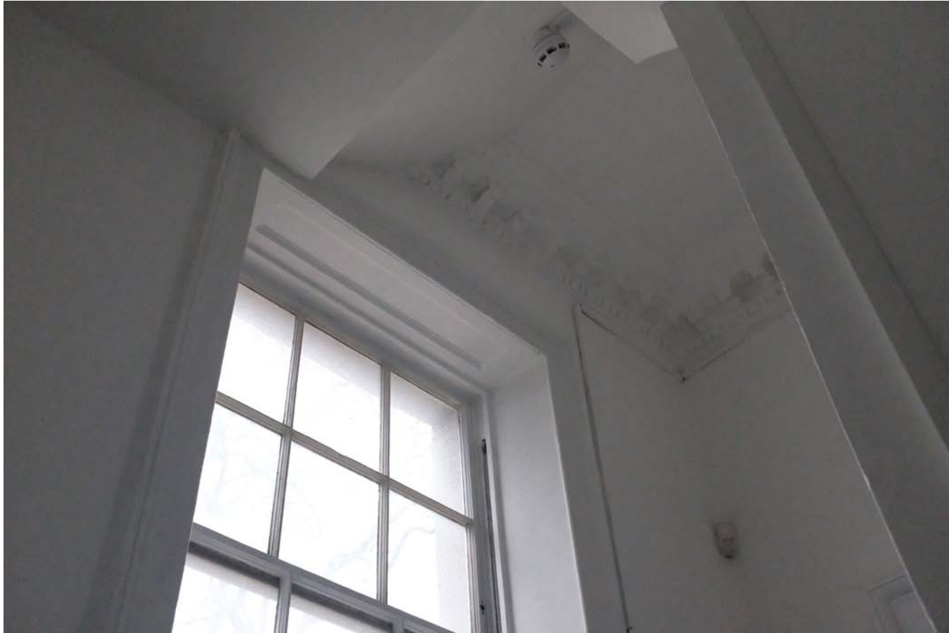
OJ. Ground to First Floor Stairwell 2985.JPG
