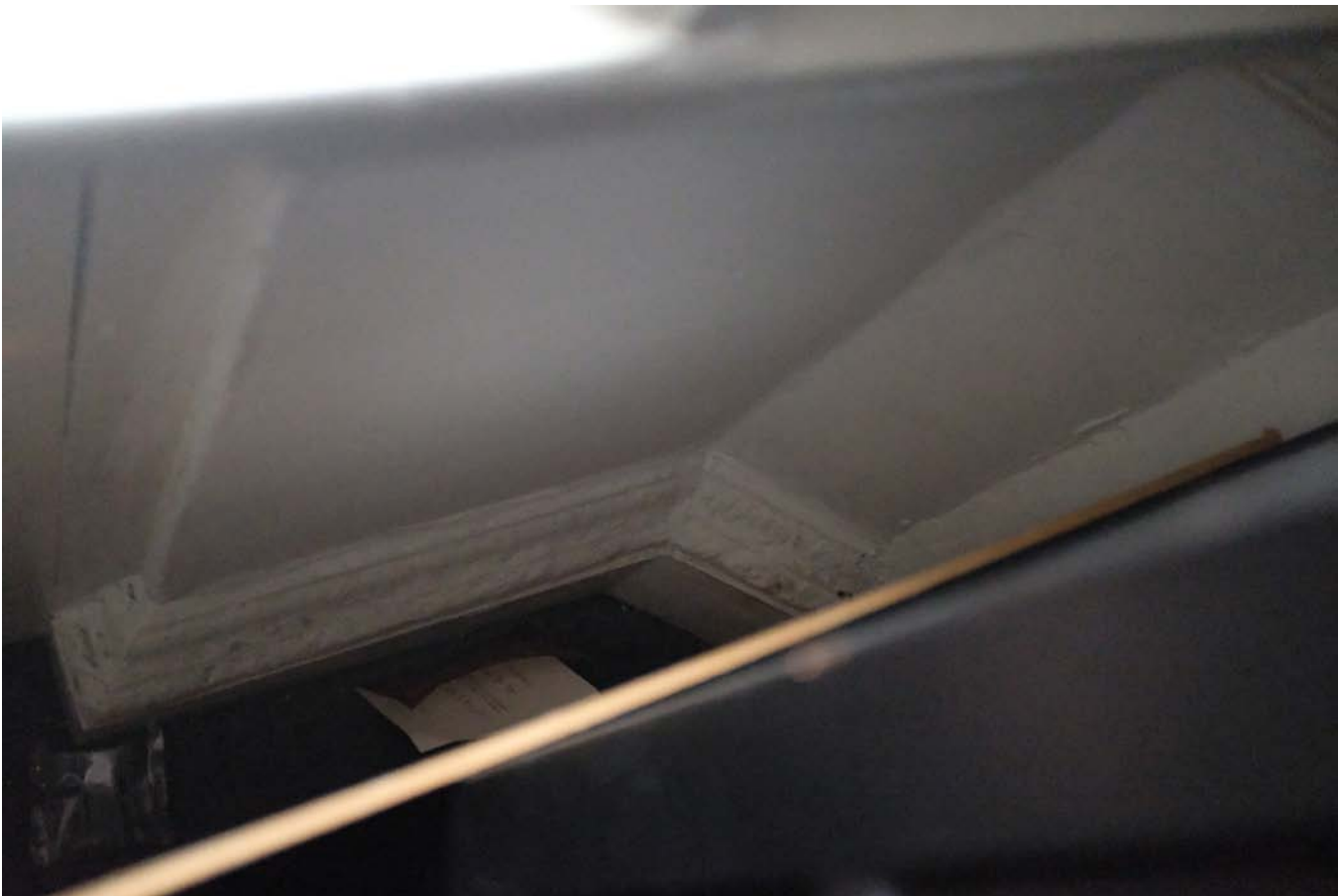
OD. Back Middle Room 2962.JPG
