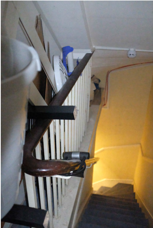
-1J. Basement to Ground Stairwell 3208.JPG
