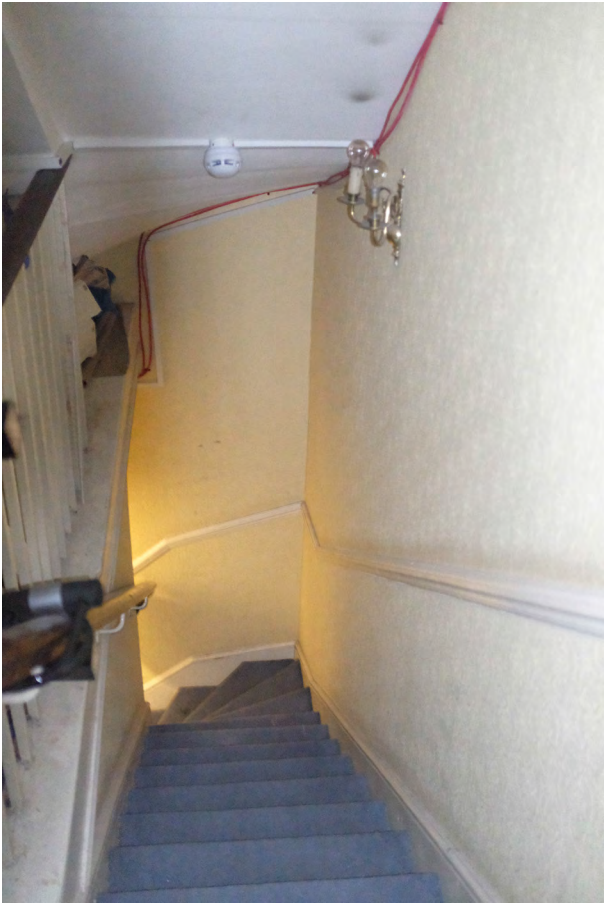
-1J. Basement to Ground Stairwell 3207.JPG
