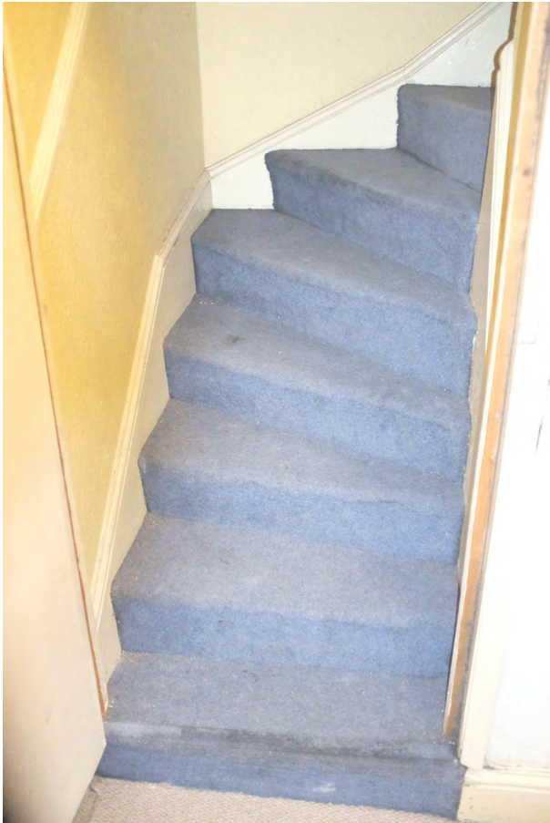
-1J. Basement to Ground Stairwell 3204.JPG
