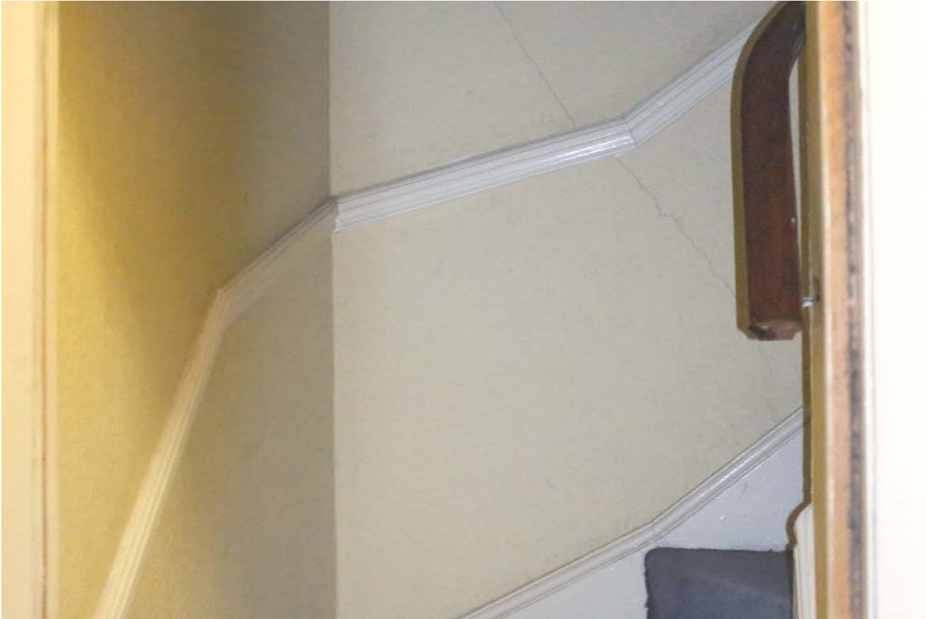
-1J. Basement to Ground Stairwell 3205.JPG
