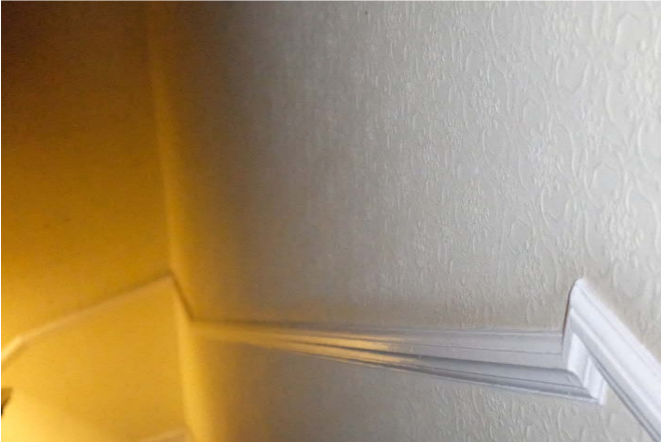
-1J. Basement to Ground Stairwell 3209.JPG
