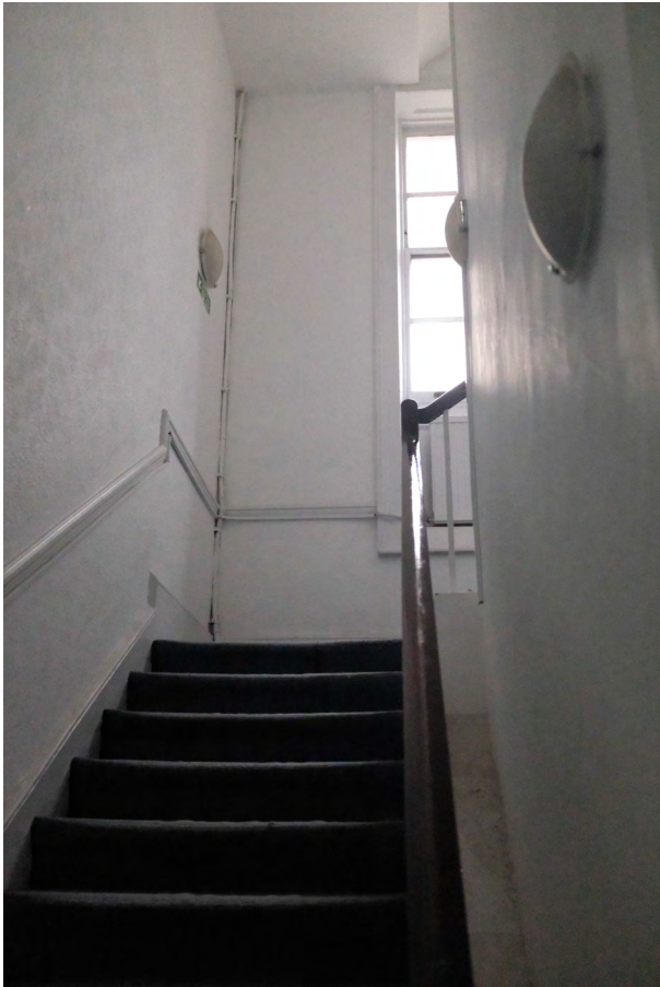
OJ. Ground to First Floor Stairwell 2984.JPG
