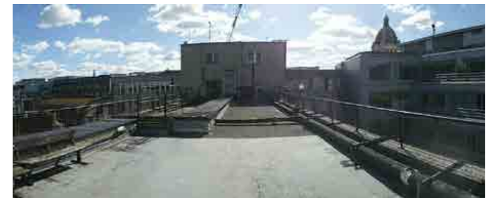
Panoramic Views of Existing Terrace.
