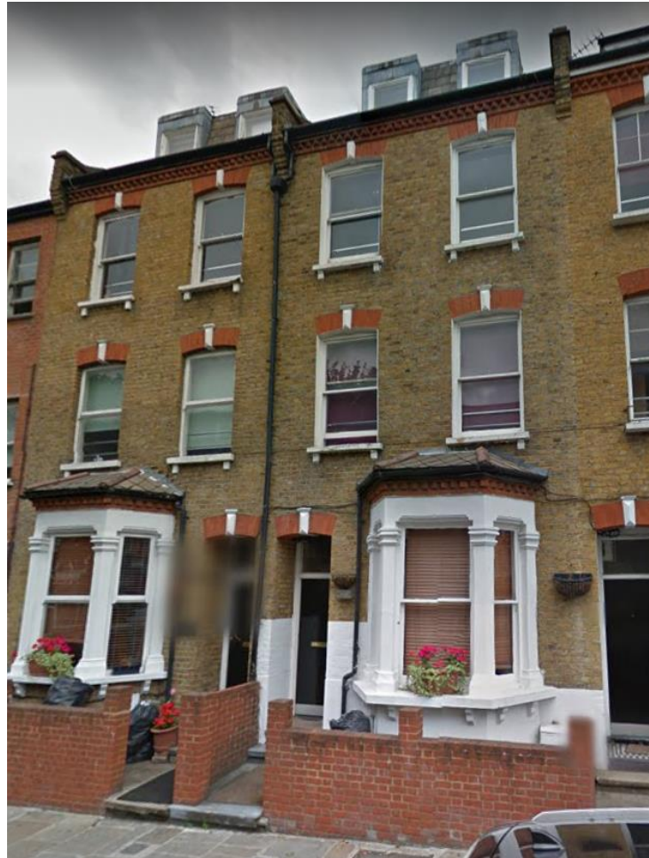
Figure 12: front of No 14 Fortess Road
