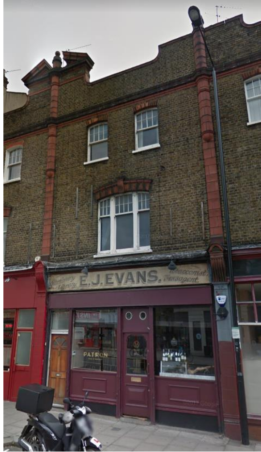
Figure 10: front of No 16 Fortess Road
