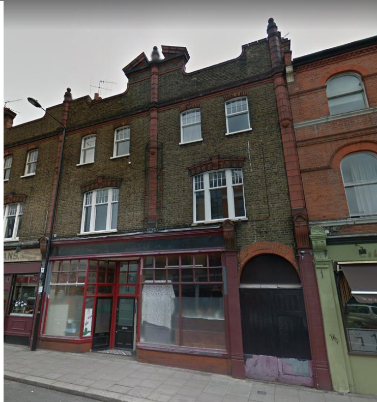
Figure 11: front of No 14 Fortess Road
