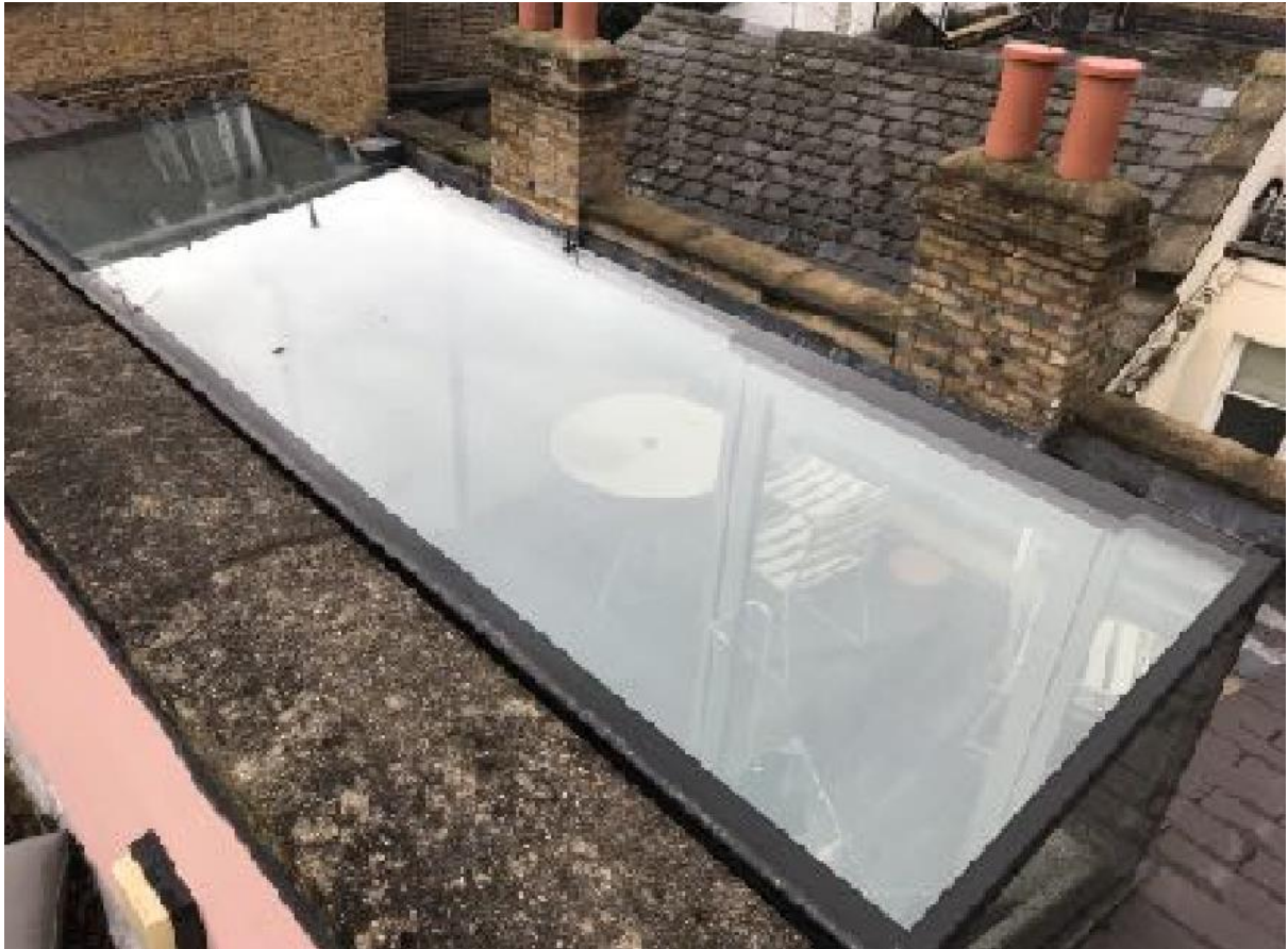
Photo 8: Glazed access roof structure at no. 5 Albert Terrace Mews
