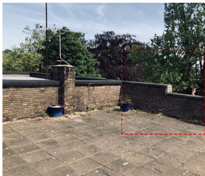
Remedial works to be carried out on the roof parapet
