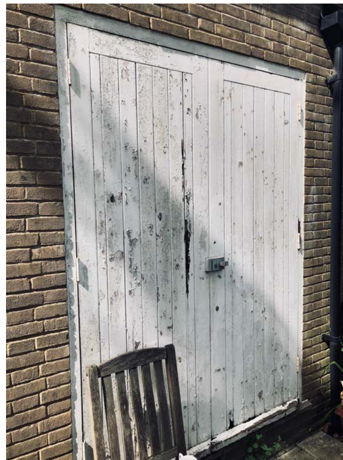
Existing Garage Door @ Rear
