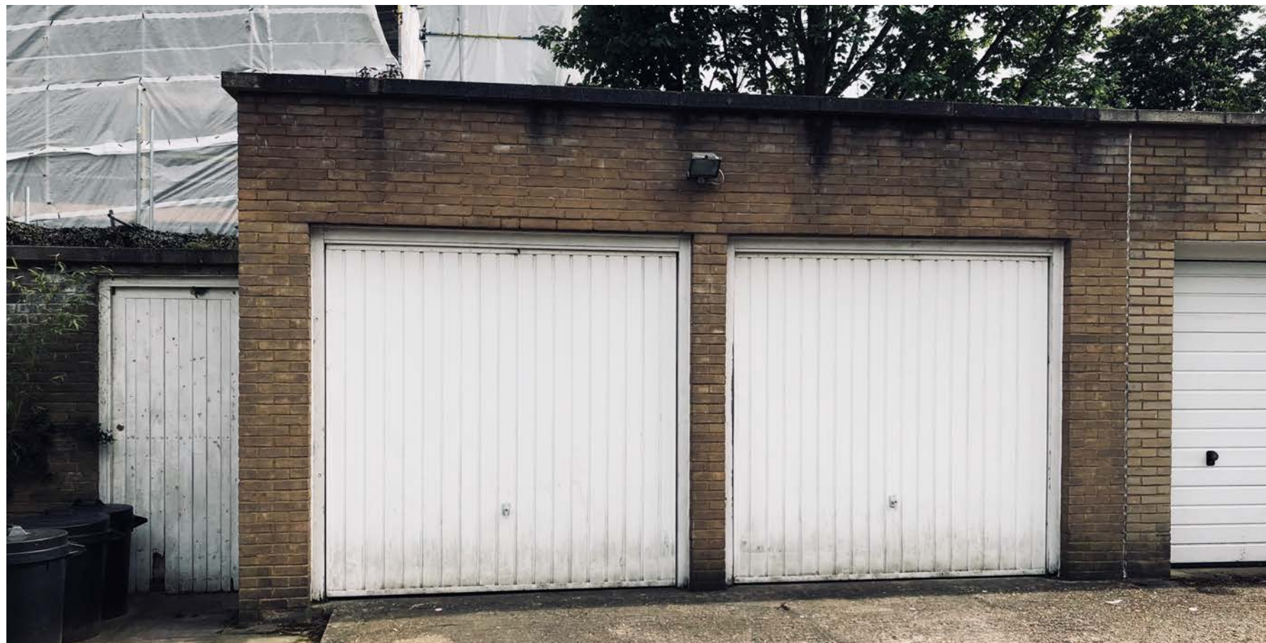
Existing Garage Doors
