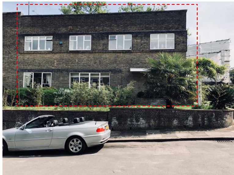
Carefully controlled acid cleaning proposed to be used to clean the brickwork
