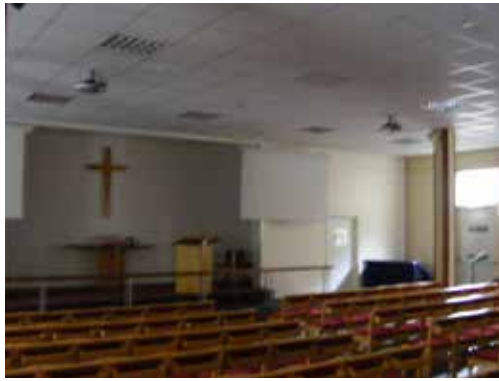
The main chapel space provides evidence of the gallery columns, although it is thought that these have been strengthened to provide the floors above. The recess on the far wall would have provided the location of the pulpit and organ above.
