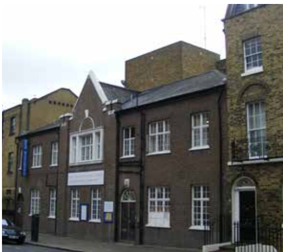
Existing frontage to Crestfield Street
