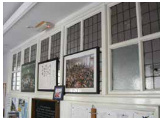
The leaded glazing between the lobby and the chapel is one of the very few remaining features - these are of late 19th century date.
