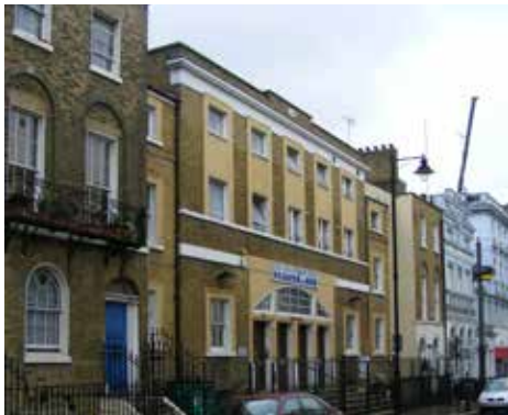
Birkenhead Street frontage, looking north. The frame of the original chapel is legible but the building is now almost residential in character.
