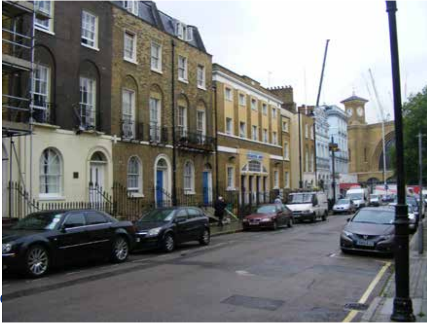
View north from Birkenhead Street, with King's Cross Station in the background
