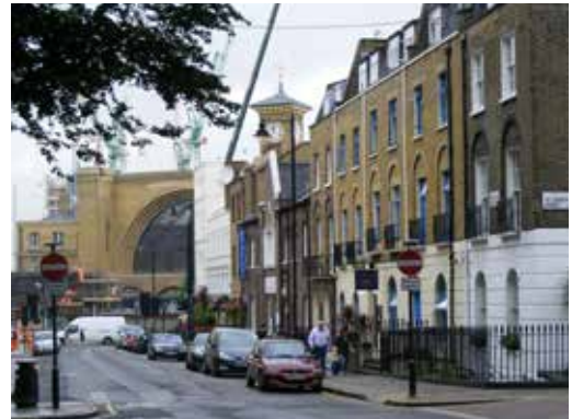
The formality of the terracing which run along Argyle Square and into Crestfield Street is broken by the Mission House. Its gable is not a strong presence but it does bring variety as Kings Cross is approached.
