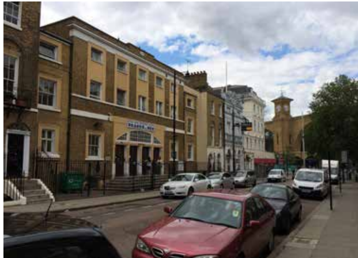
Existing frontage to Birkenhead Street
