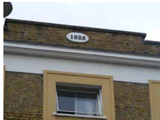
The 1825 datestone has been planted on an altered parapet which used to form part of the front pediment, removed when the roof was taken down to create the top floor flats.
