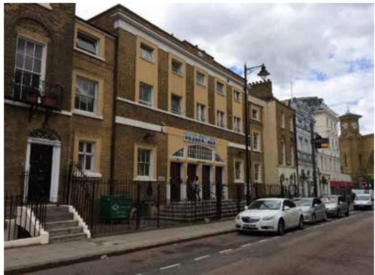
The Birkenhead Street frontage is a poor residential conversion of the former chapel
