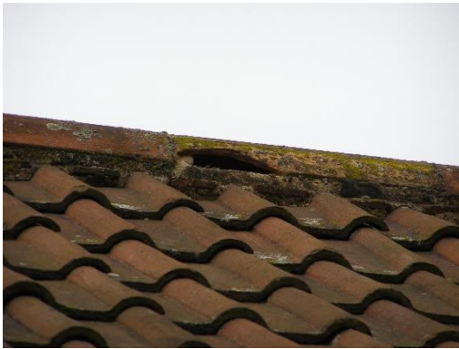
Hole and missing section of ridge tile in building 2
