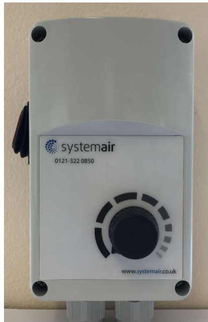
Fig 1 – Fan control set at full speed (Typical speed controllers shown)
