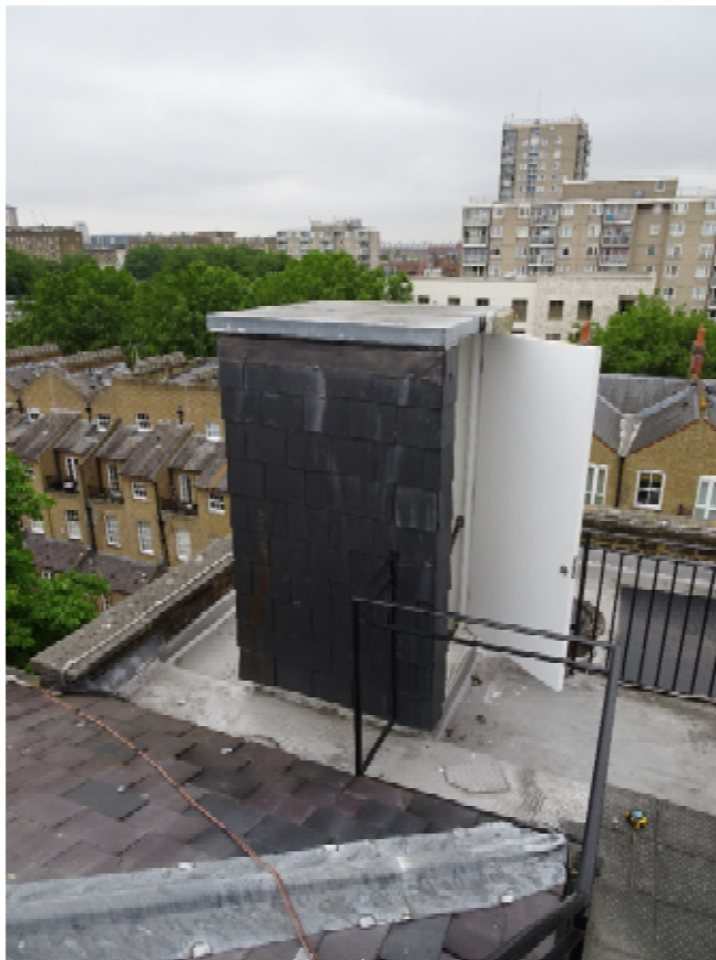
2) Existing access stairs to the rear of the property
