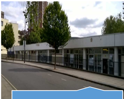
Existing Charlie Ratchford center directly opposite Site 1
