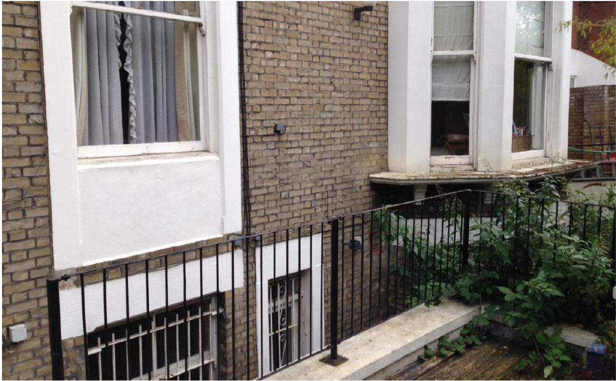
6. Rear view of No. 35 Belsize Avenue (neighbouring pair to No.33), showing scale of light well.
