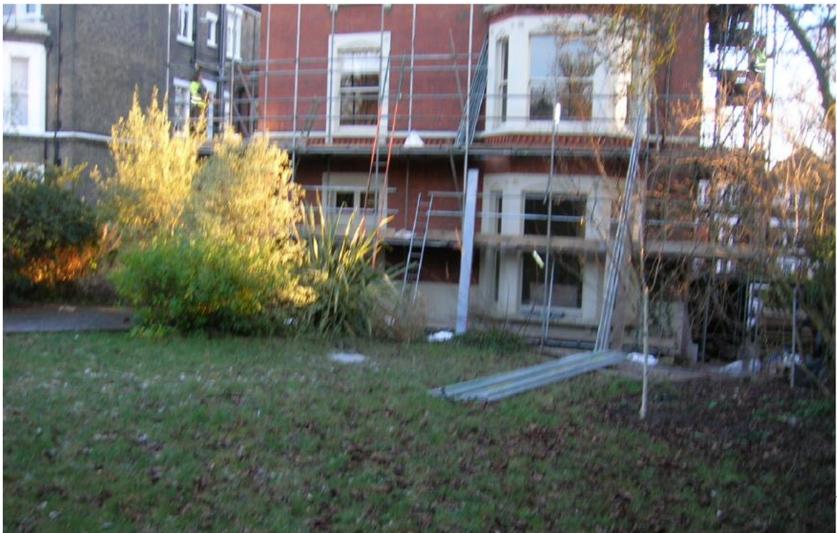
7. Rear view of 33 Belsize Avenue in 2009, prior to garden excavation.
