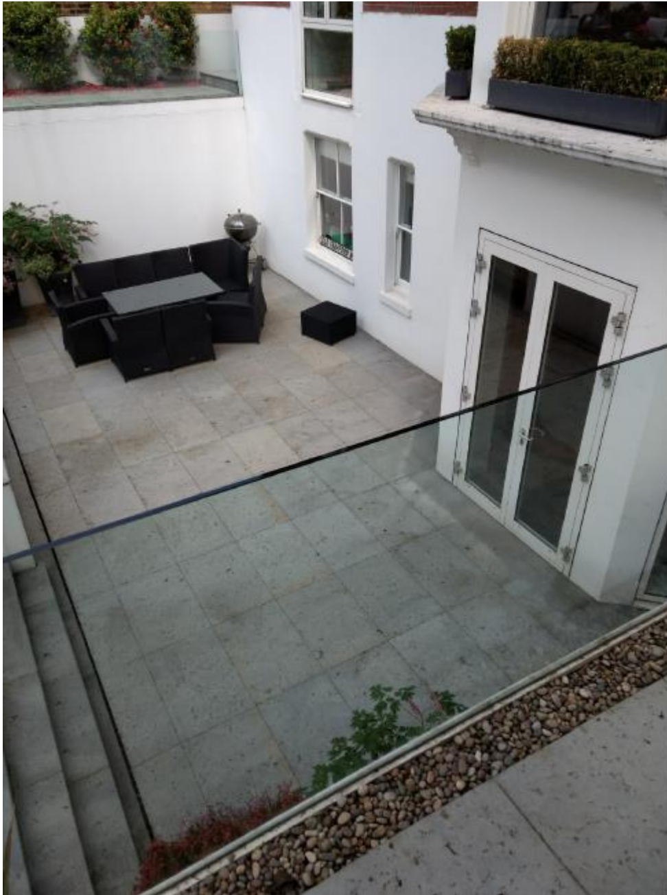
3. Existing rear sunken patio.
