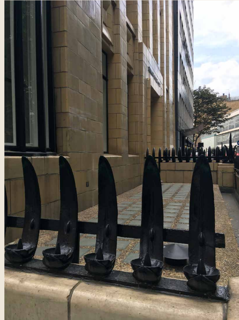
6.4.A Existing lightwell 'lid' from corner of Red Lion Square and Dane Street
