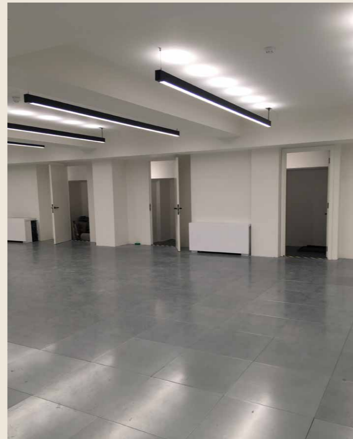
5.3.F Lower ground floor enclosed pavement lights to north
