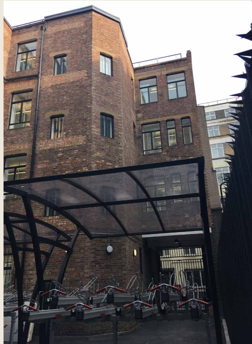
5.2.M View of southern building from service yard
