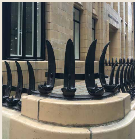
5.2.B Iron railings
