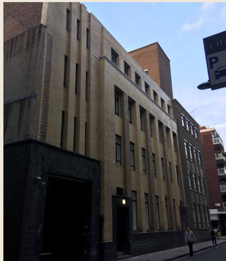
5.2.K Eagle Street facade - looking towards Dane Street
