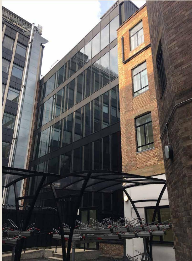
5.2.L East facade to service yard
