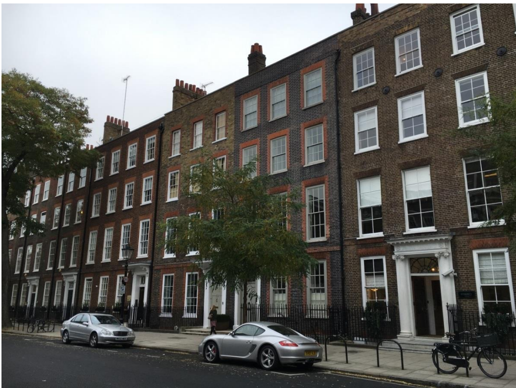
Figure 3.39: Bedford Row (Terraced townhouses largely dating from the late 17 th and early 18 th century)
