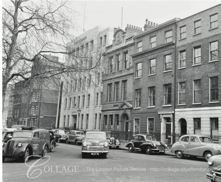
Figure 3.28: Archive Photograph dated 1956 39 (above entrance lettering “Austin Reed Ltd”)
