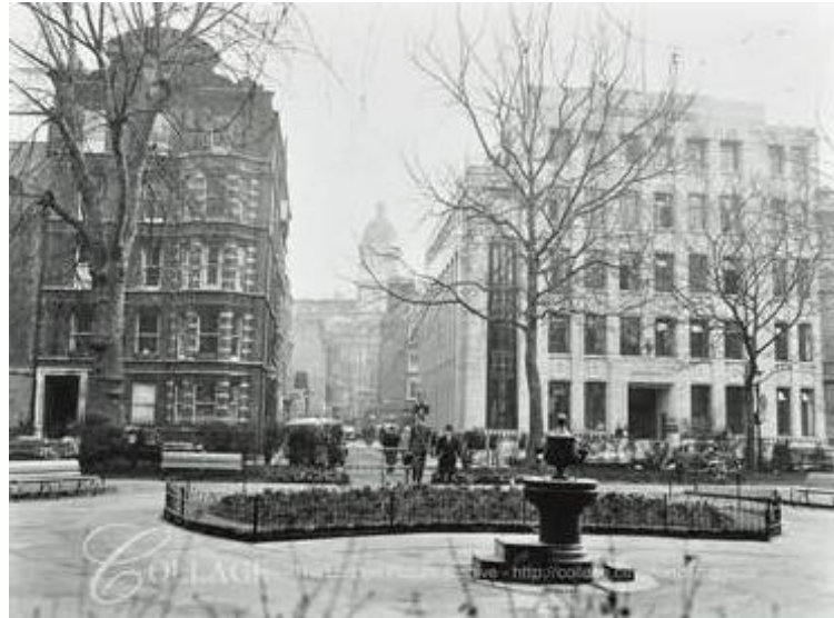
Figure 3.10: Archive Photograph dated 1956 26 (above entrance lettering “Austin Reed Ltd”)
