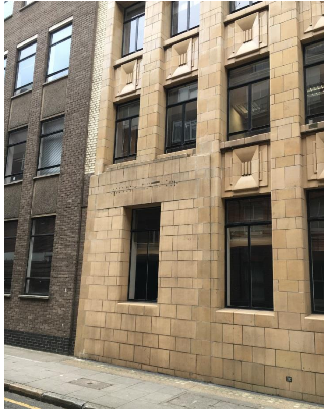
Figure 3.17: Typical fenestration material and design – showing similarity of existing units to interwar and 1950s elements, as well as matching later 20 th century unit to former doorway to Dane Street
