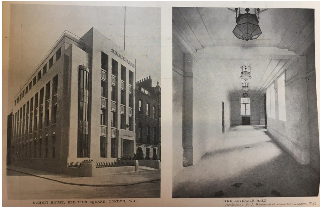
Figure 3.2: Illustrations - External and interior (Entrance Hall) Summit House as built in 1925 16
