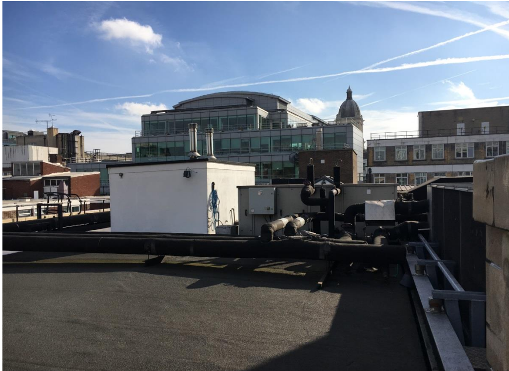
Figure 3.18: Roof Level (with modern plant / service elements)
