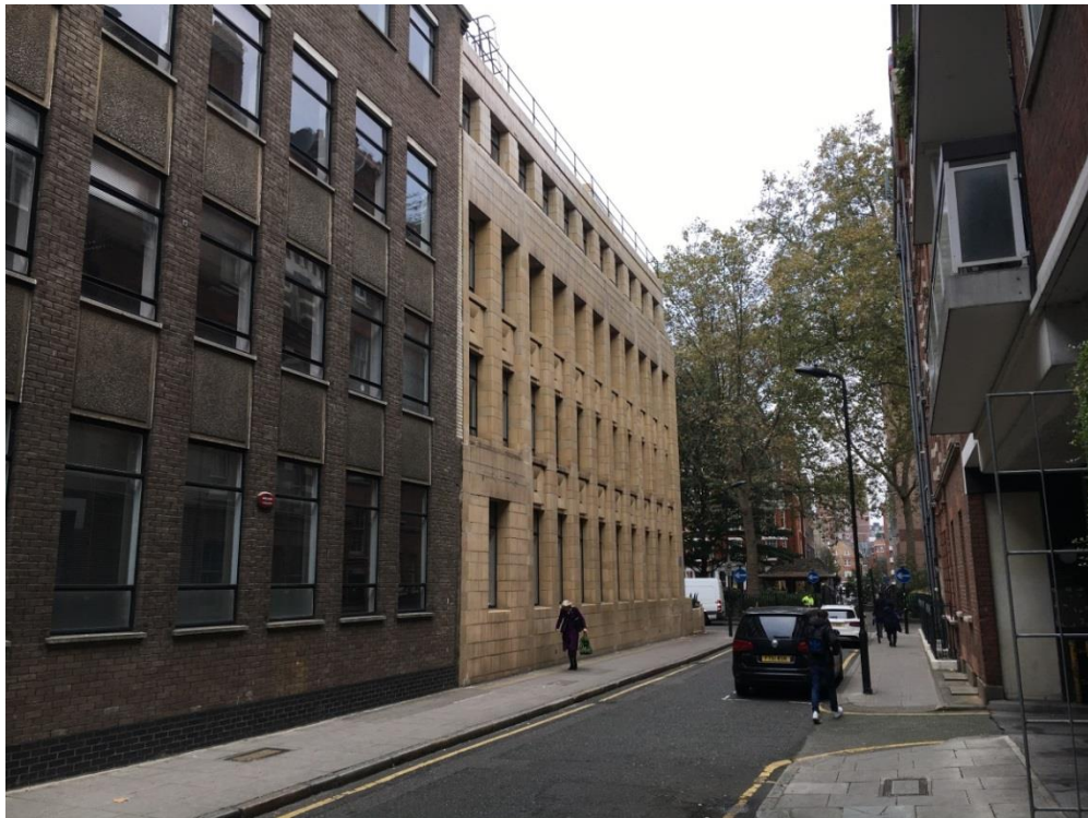
Figure 3.15: Dane Street Elevation (Clear distinction between original 1920s office building and later 1950s warehouse extension)
