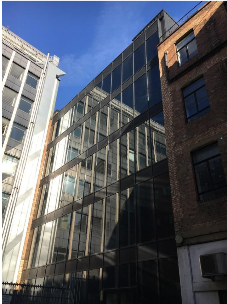
Figure 3.8: Rear (East) Elevation of Summit House to Yorkshire Grey Yard (Glazed extension dating from 2000s)
