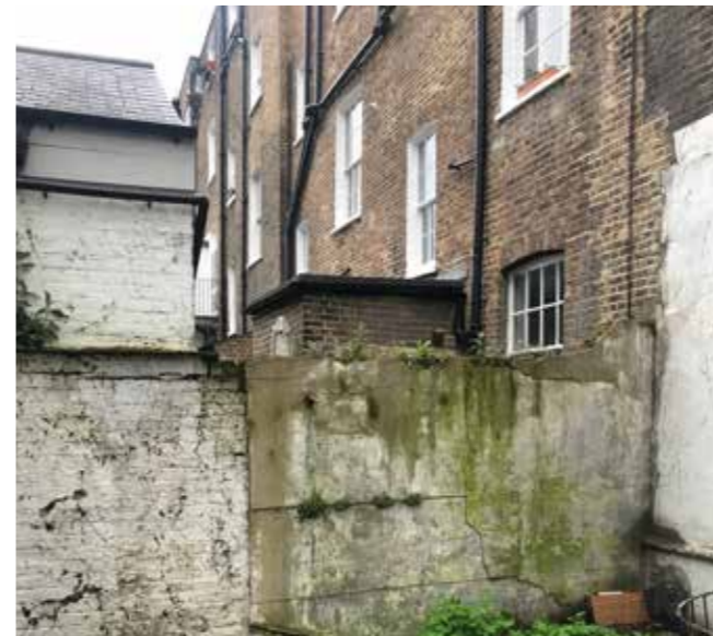
Boundary wall to no.5
