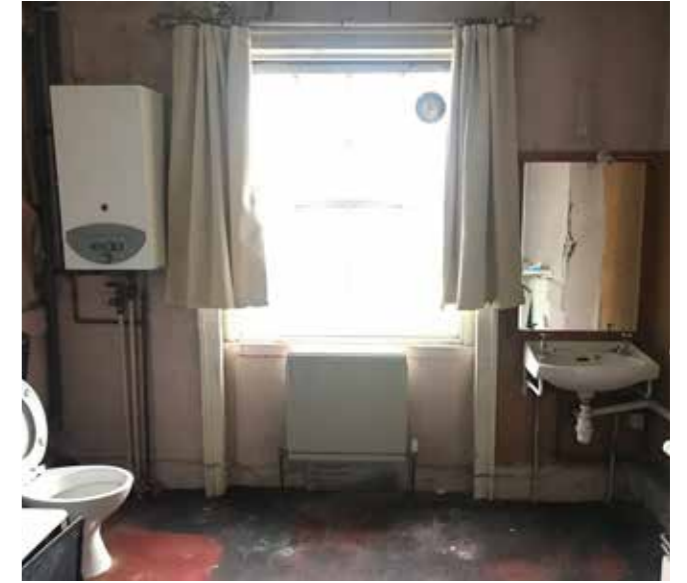
Second floor bathroom
