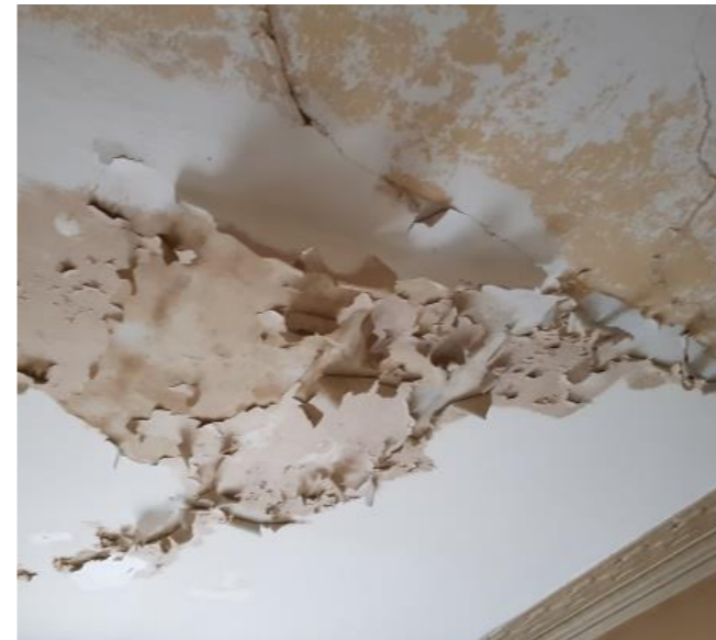
Ceiling to first floor rear room
