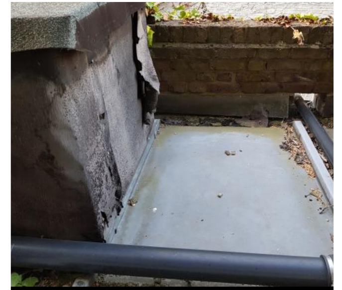
Cold water tank to closet wing roof
