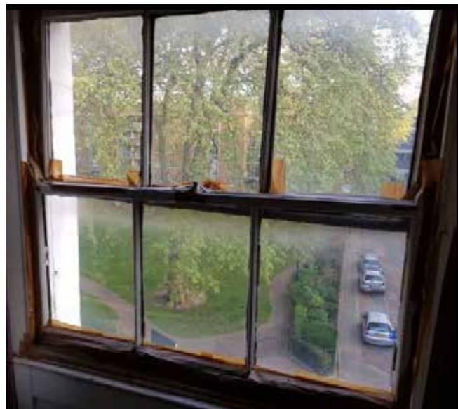
Window to front right bedroom at fourth floor
