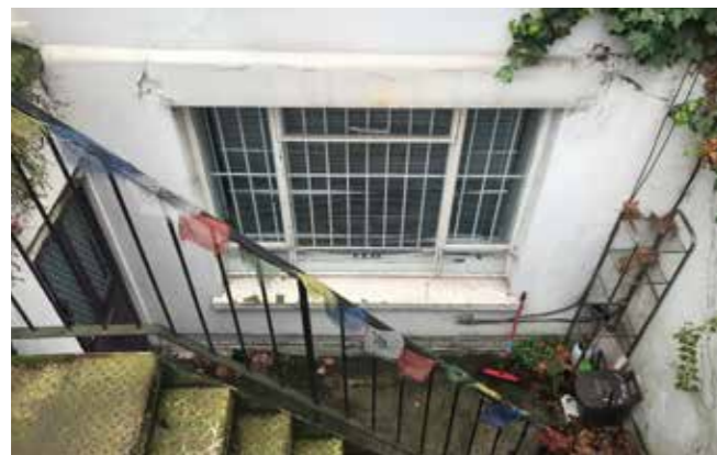
Front lightwell with crittal window to lower ground floor
