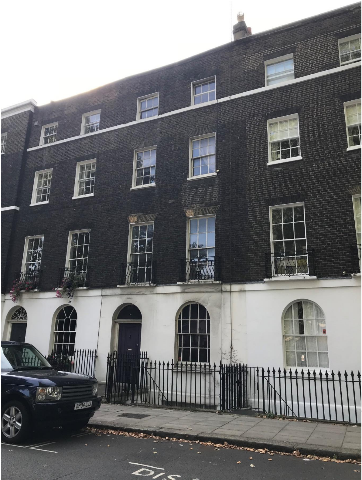
Figure 6 – 4 Regent Square Frontage, Site Visit 2018
