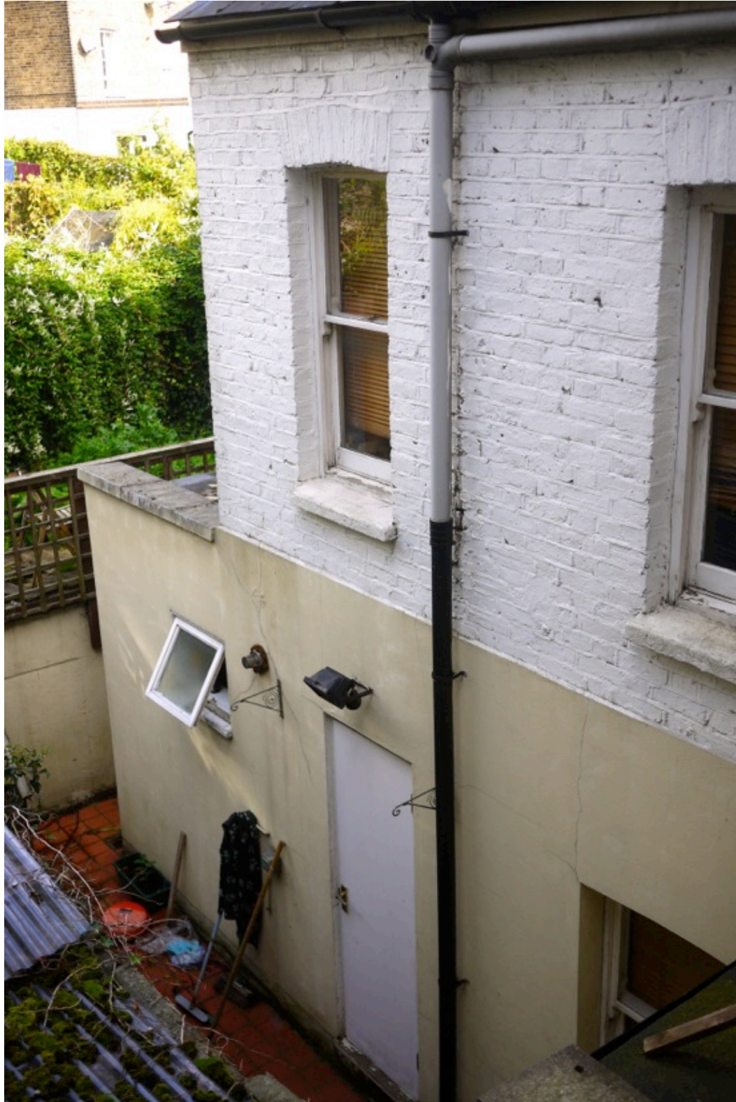
Rear of no. 47 facing rear extension of no.45
